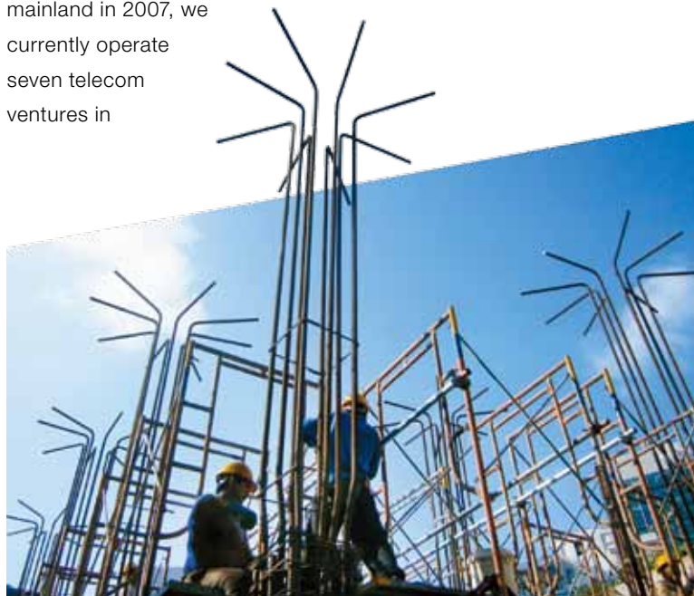
Construction of the Bowen Drive Salt Water Pumping Station, the Magazine Gap Road Salt Water Service Reservoir and associated works by U-Tech for the Water Supplies Department.
