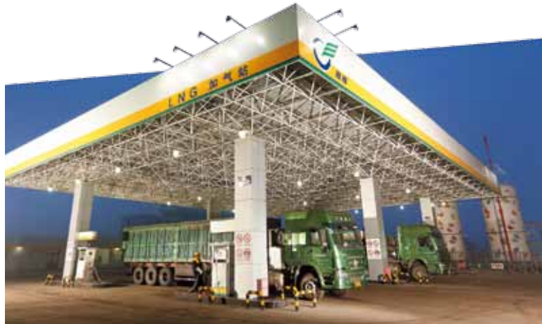
A liquefied natural gas filling station for heavy-duty trucks in Chiping, Shandong province.
