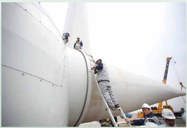
The generator of the 6MW double-fed offshore WTG 6MW海 上雙饋風電機組發電機
