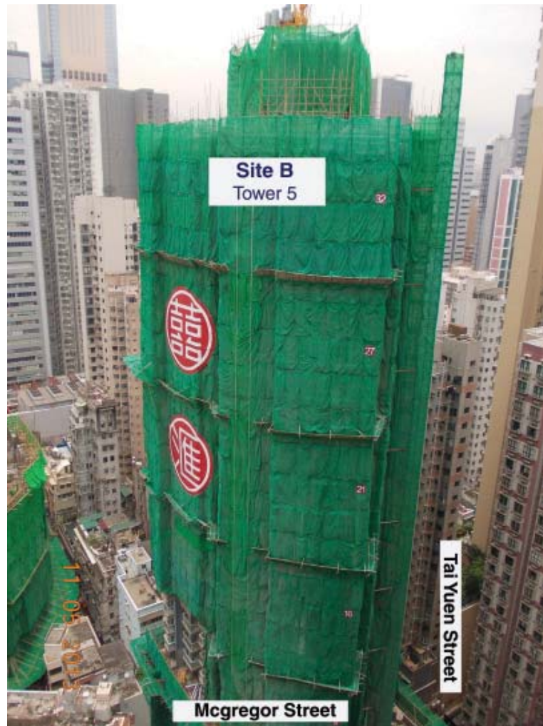
Note: Site B of 200 Queen's Road East Project (as at 11 May 2013)
