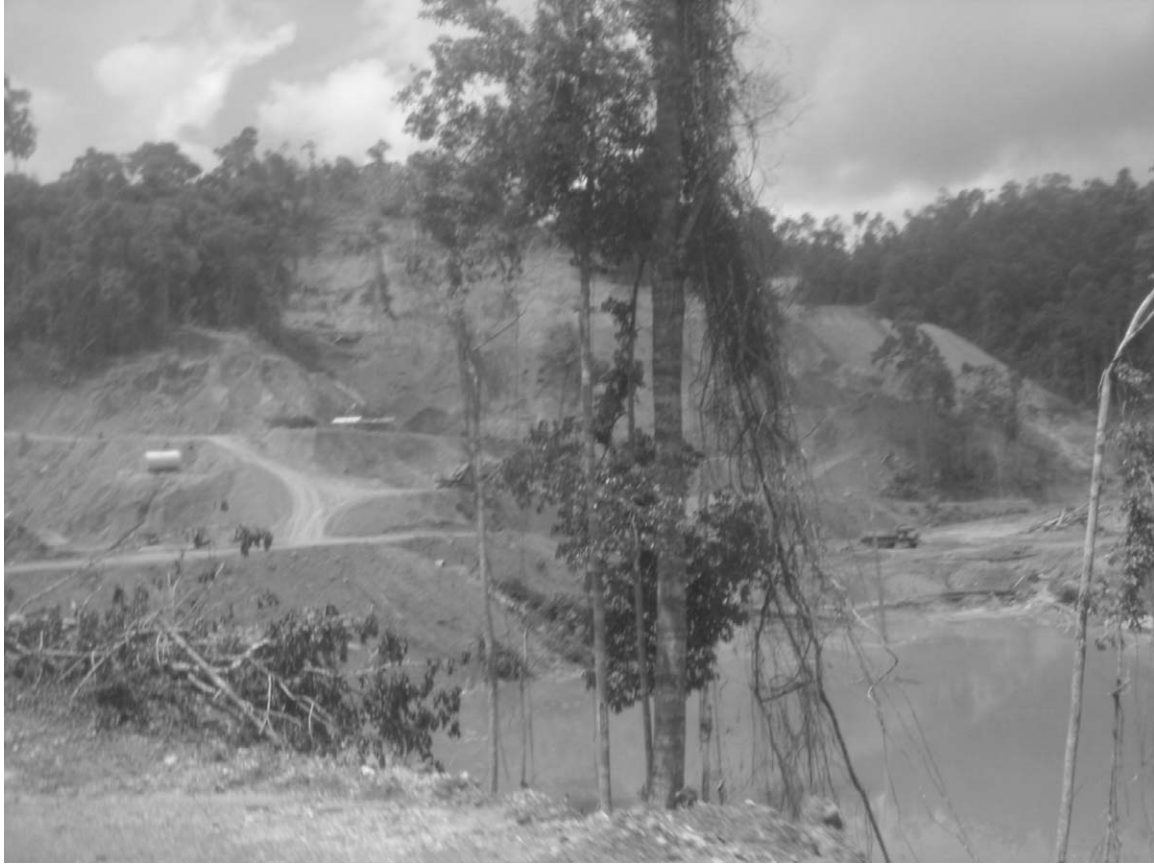
Photo 5: Retention pond for runoff and drained waters
