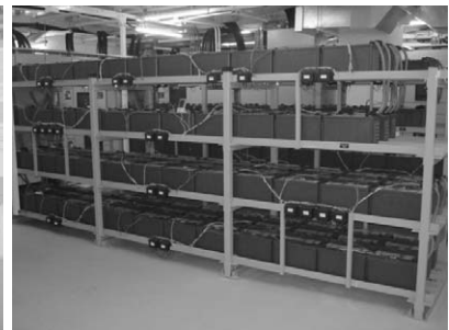
Batteries for UPS systems
