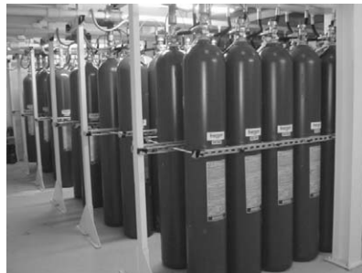
Storage of inergen gas
