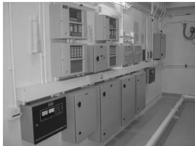
Panel of inergen system for monitoring the operation of fire suppression system
