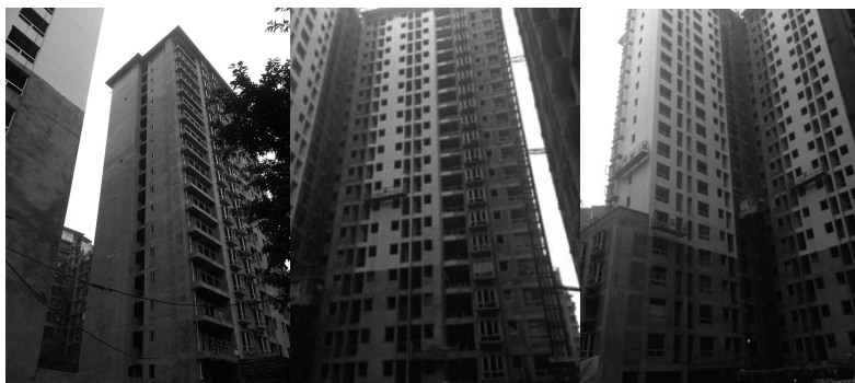
Construction Site of ShuXiangYuan (書香苑)
