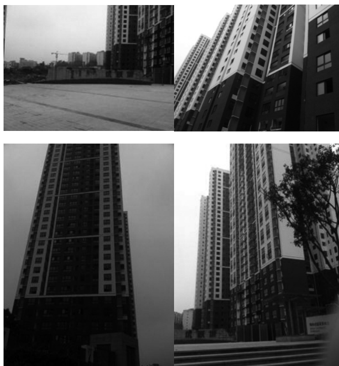
Construction Site of TongJingYueCheng (同景•躍城)
