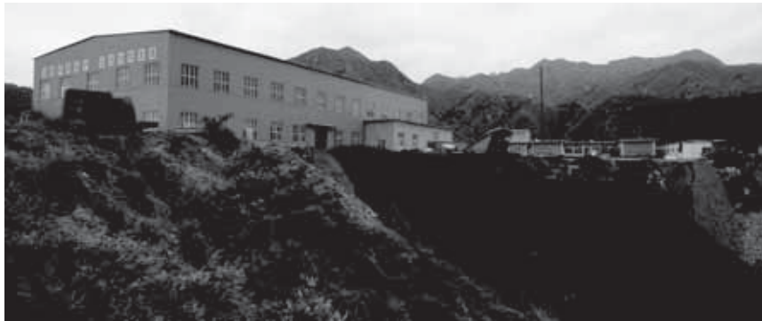
Figure 8-8: Tailings' Dewatering Facility and Discharge after Dewatering of Chengzigou TSF
