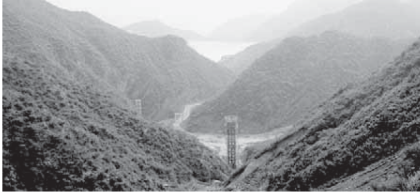
Figure 8-7: Overview of Xiaomazong Tailing Dam
