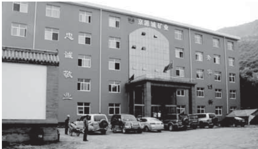
Figure 12-2: The Office Building of Jingyuancheng Mining
