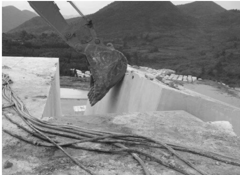
Figure 8.10. Excavator pushing for large rectangular stone overturning
