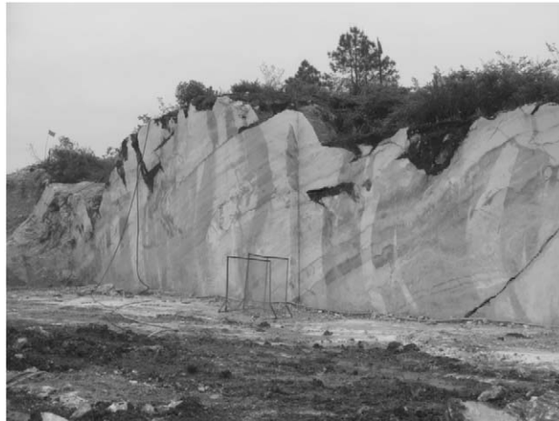
Figure 8.4. Top soil and weathered rock zone of the North #1 mining area
