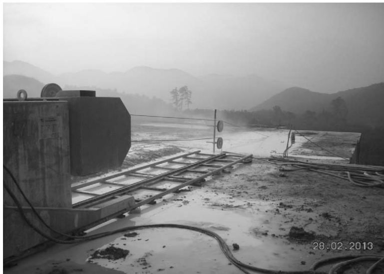
Figure 8.7. Vertical cutting by a diamond wire cutting machine
