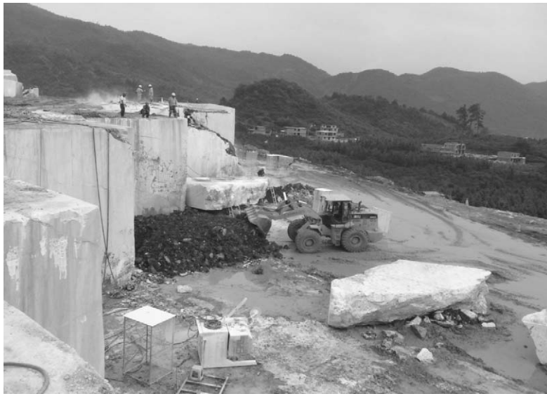
Figure 8.8. Prepare the cushion layer for large rectangular stone overturning
