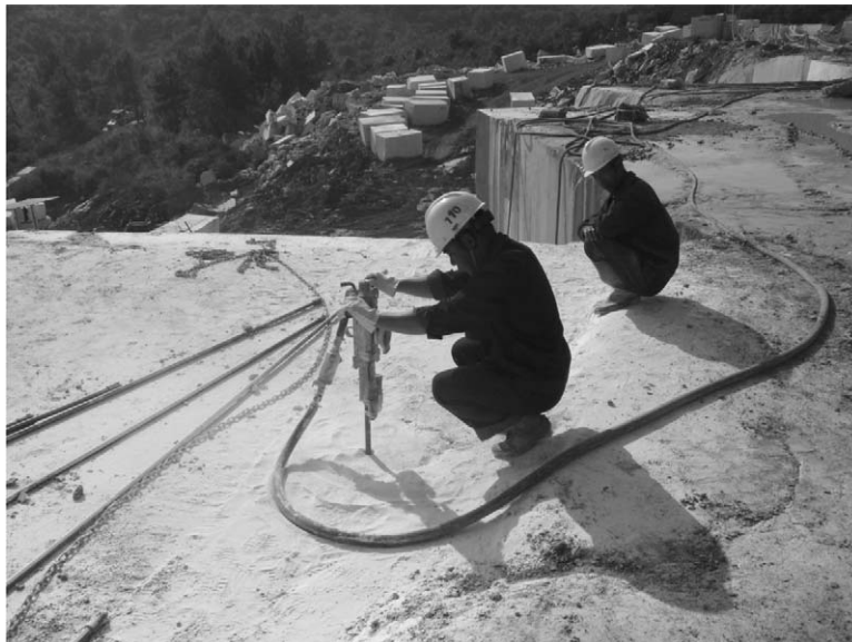
Figure 8.5. Vertical hole drilling using a jackleg drill
