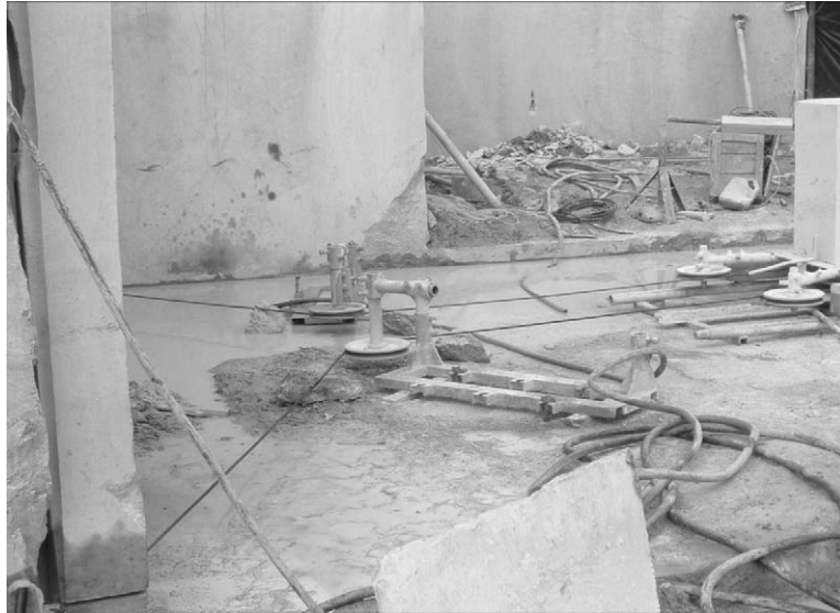
Figure 8.6. Horizontal cutting by a diamond belt saw
