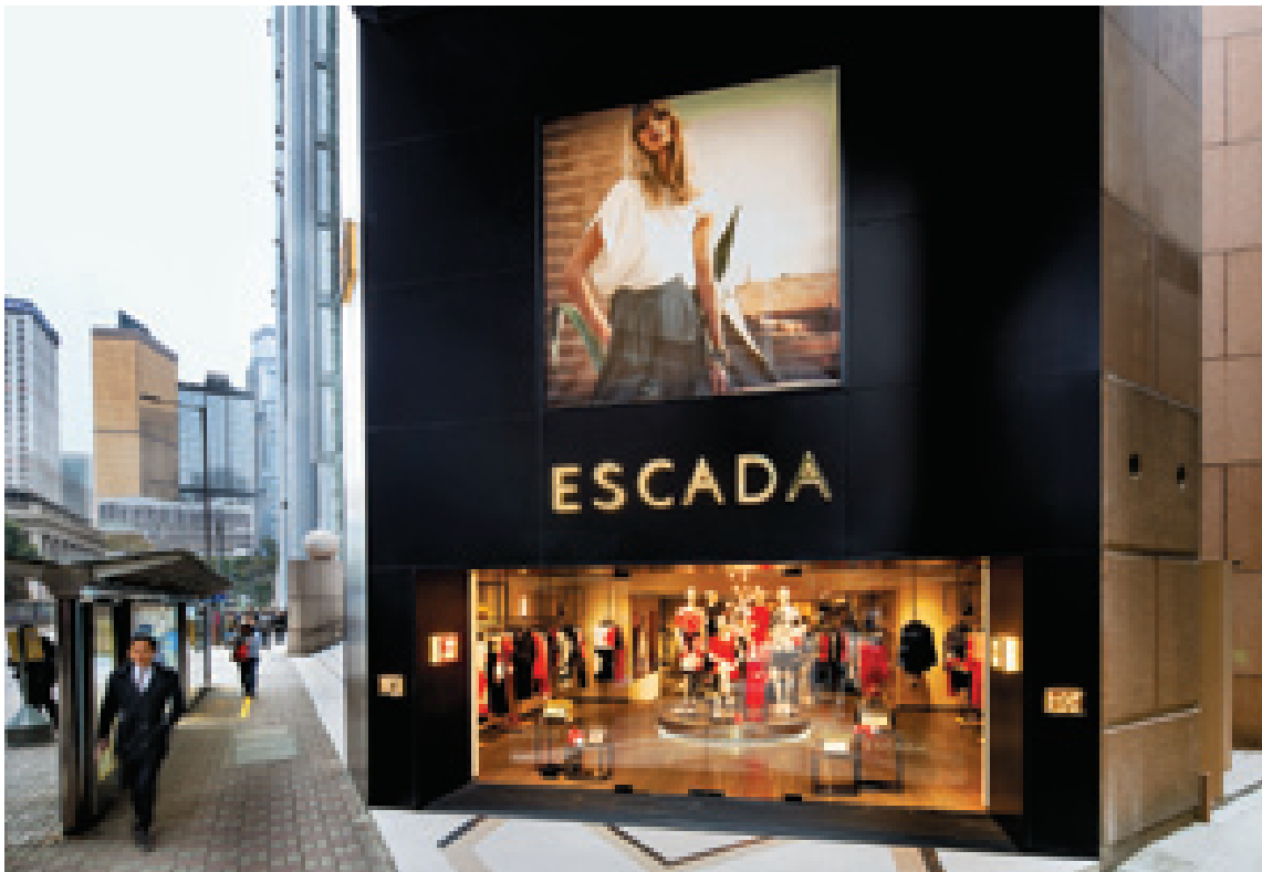
在渣打銀行大廈開店之高檔品牌 Luxury brands open shops at the Standard Chartered Bank Building
