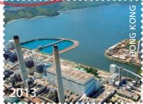
Lamma Power Station Coal-fired: 2,500 MW Gas-fired combined cycle gas turbine: 680 MW Oil-fired gas turbine: 555 MW Solar: 1 MW Wind turbine: 800 kW Interest: 49.9%
