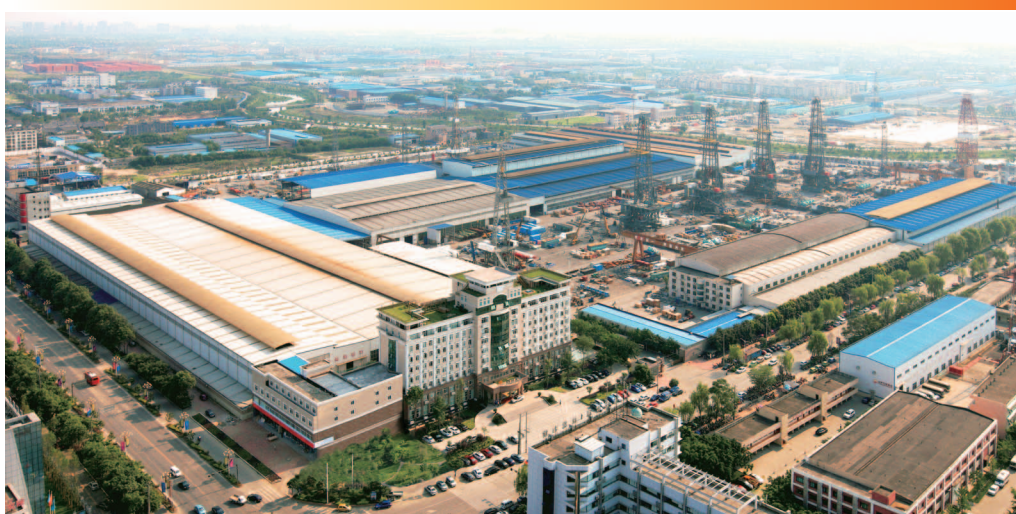
Honghua Group's land drilling rig production base — one of the largest land drilling rig production facilities in the world.
