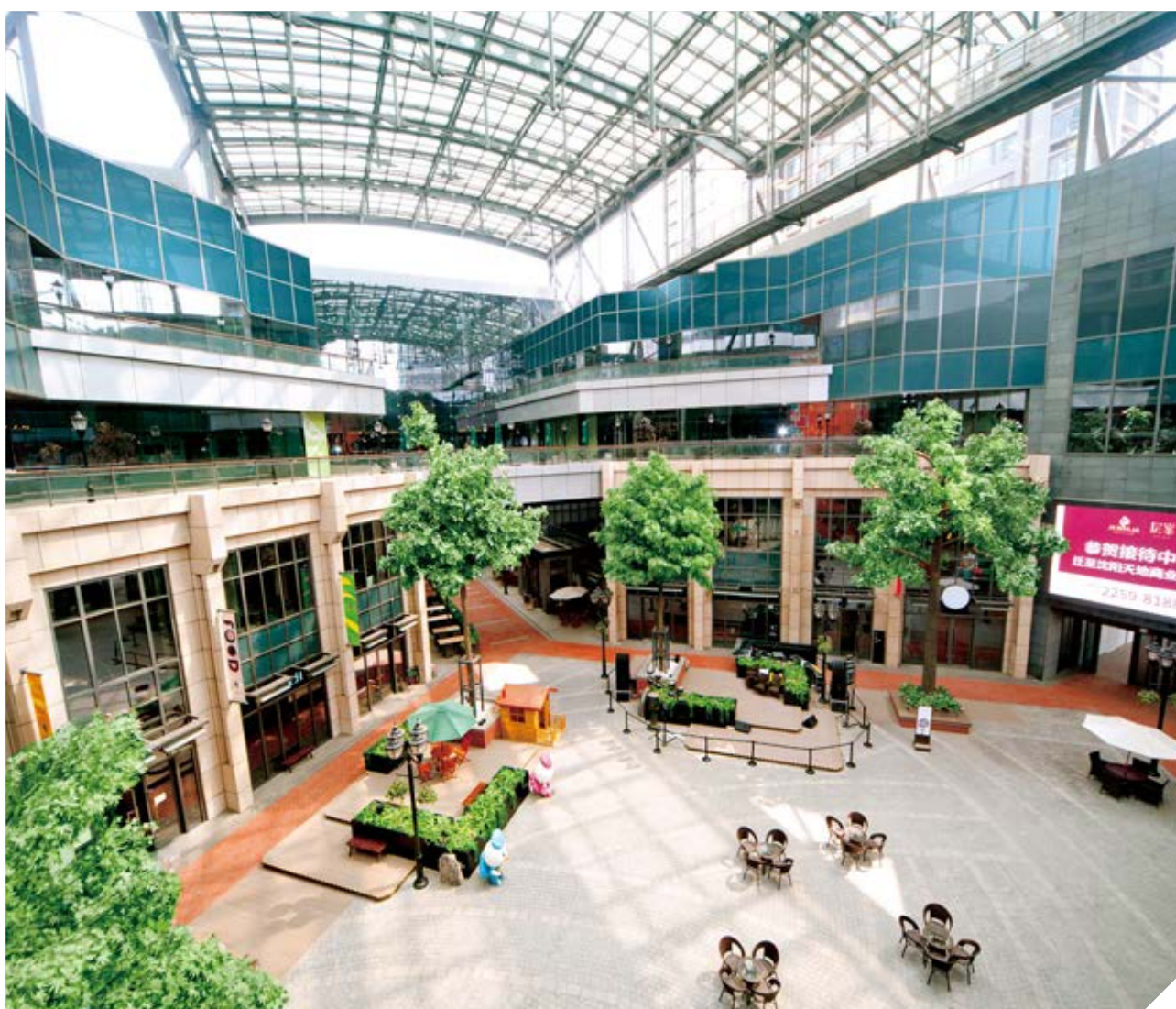
Shenyang Project Phase I
