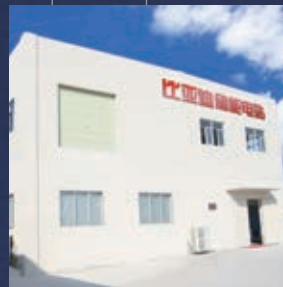
■ Energy Storage Station
