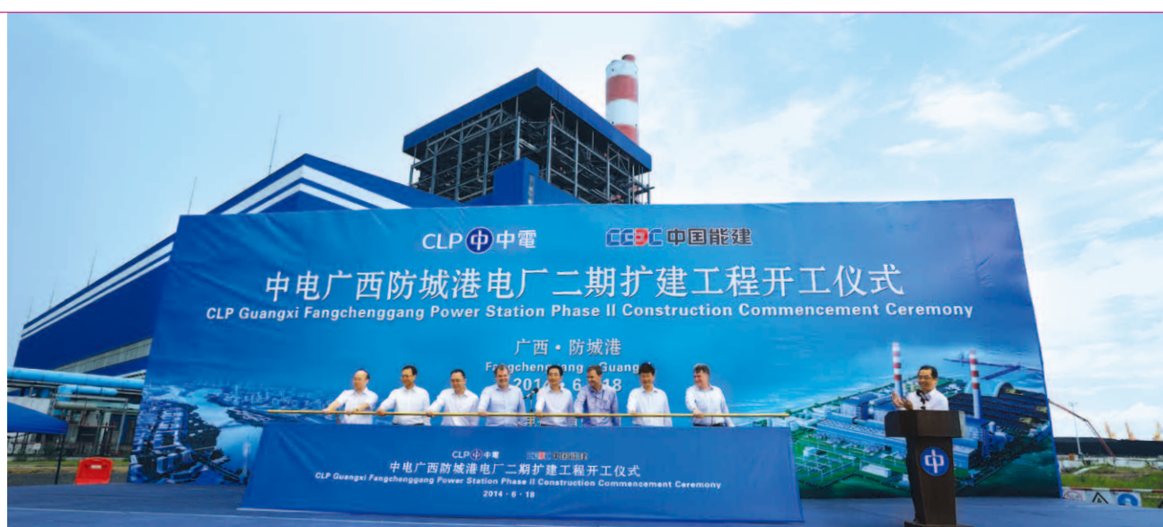
Construction of Fangchenggang Power Station Phase II commences in June 2014
