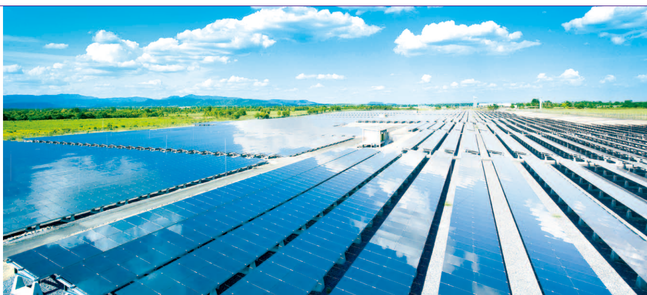
Lopburi Solar Farm enters second year of full operation
