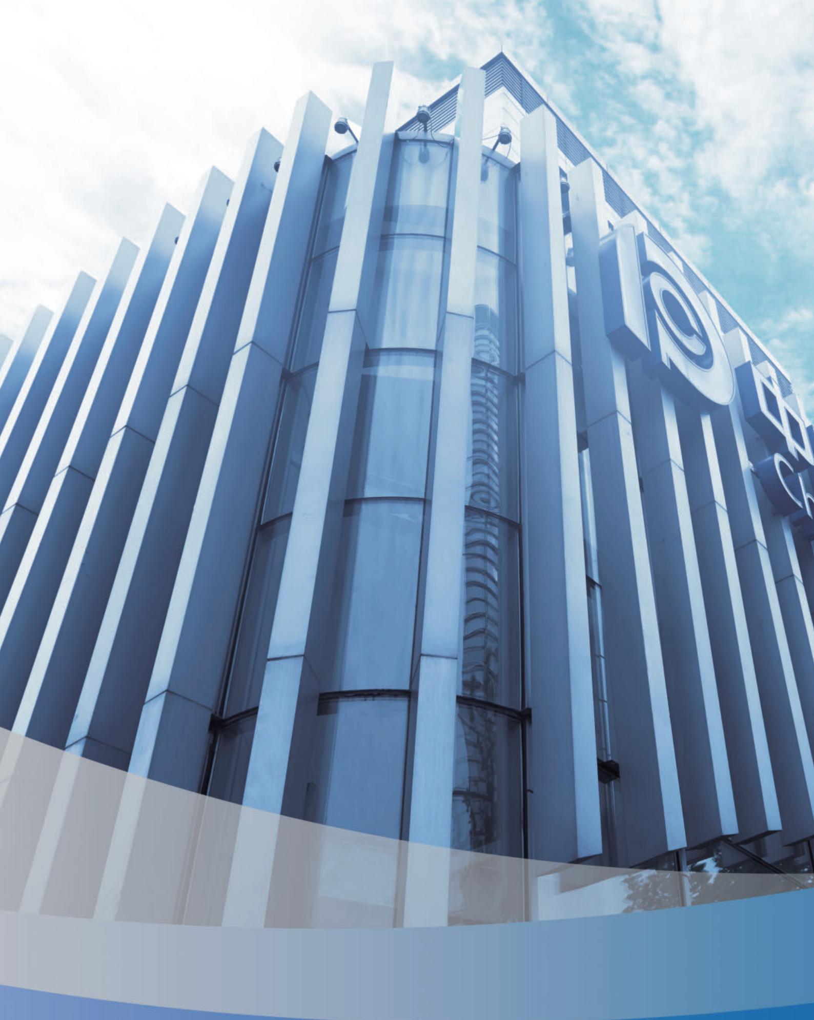
CPIC Office Building on Guilin Road
