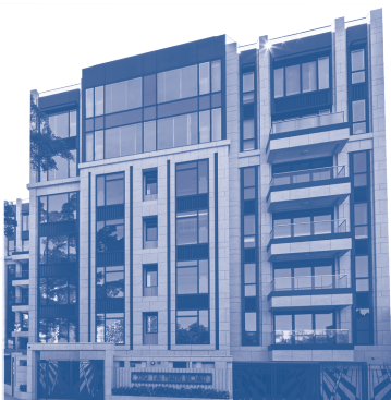
Cover Photo 335 - 339 Tai Hang Road, Hong Kong
