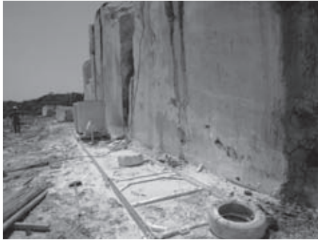
The horizontal plane of the marble rock is cut with diamond wire saw.
