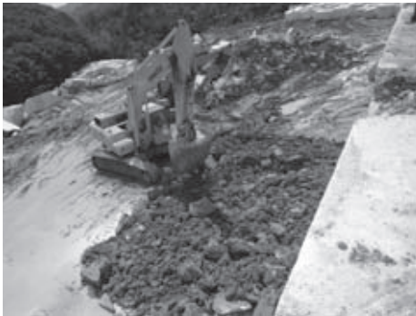
A cushion layer made up of crushed stone and soil is prepared.
