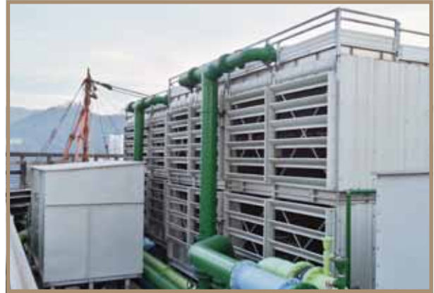
Replacement of Chiller System
