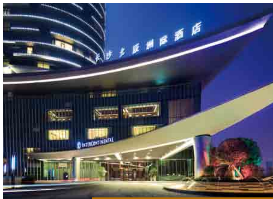
Main entrance of InterContinental Changsha North Star at night
