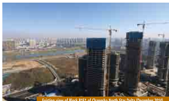
Existing view of Block B1E1 of Changsha North Star Delta (December 2014)
