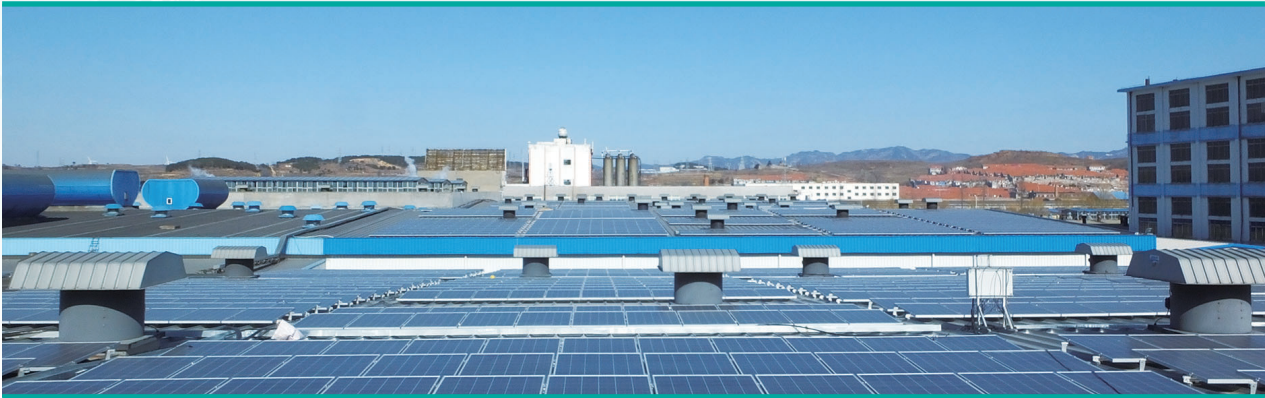
A section of Rongcheng distributed solar station
