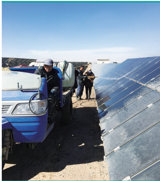
Module clean in progress at Qinghai solar farm
