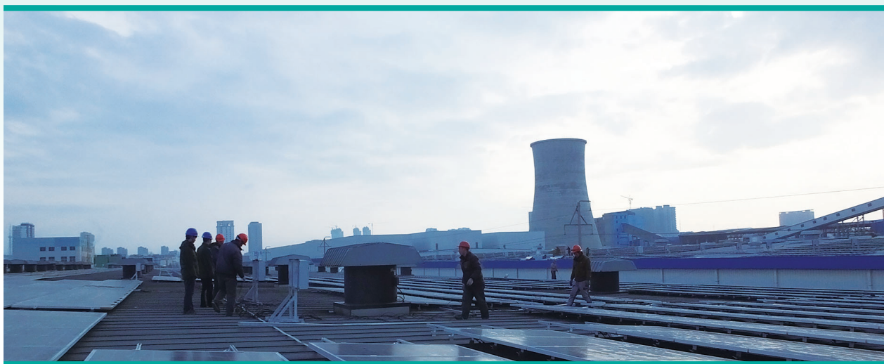
Rongcheng distributed solar station under construction
