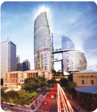
Queen's Wharf Brisbane Project
