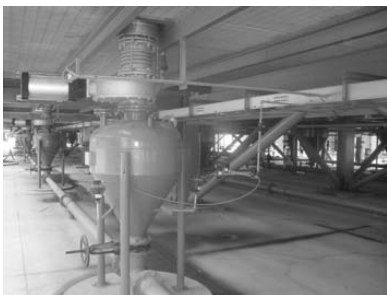
Pneumatic ash conveying system (氣力輸灰系統)
