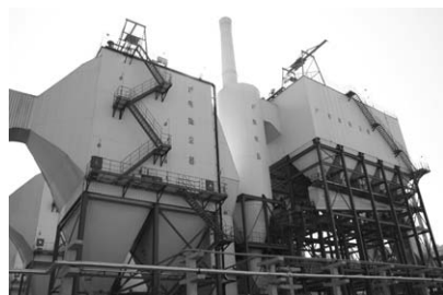
Semi-dry desulfurisation with circulating fluidised bed (循環流化床半乾法脫硫)
