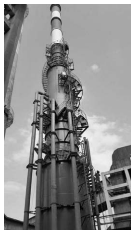
Lime-gypsum wet fuel gas desulfurisation (石灰—石膏濕法燃氣脫硫)
