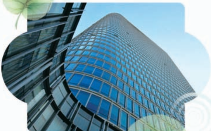
Shanghai China Fortune Tower
