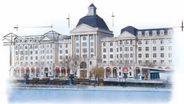
City Plaza (Tianjin)
