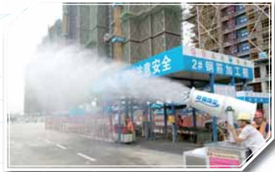
Water sprays to prevent dust at construction site 施工現場霧化降塵
