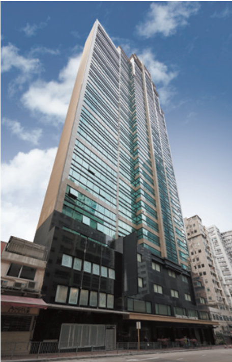
Empire Hotel Causeway Bay and the adjacent new hotel
