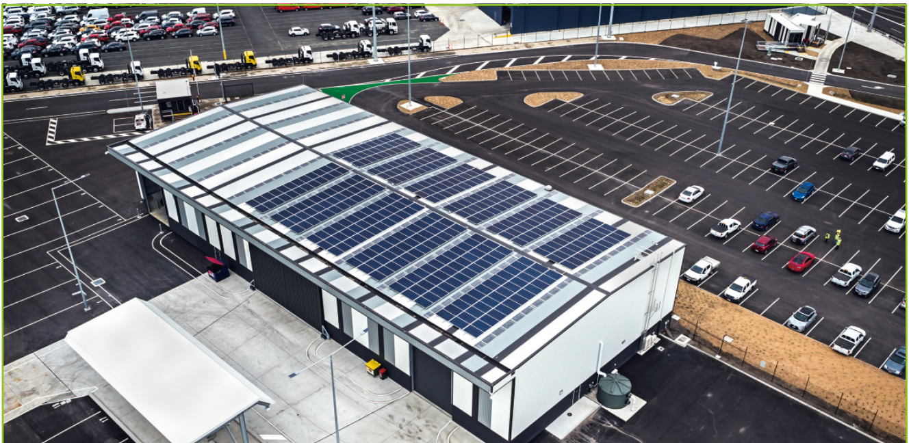
EnergyAustralia provides innovative solar power solution to MIRRAT, the largest automotive terminal in Australia
