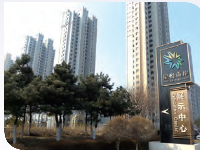
Facade of Residential Towers 住宅外景
