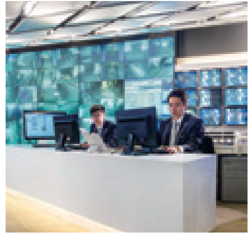
Seasoned staff and regular system improvements ensure peace of mind and comfort
