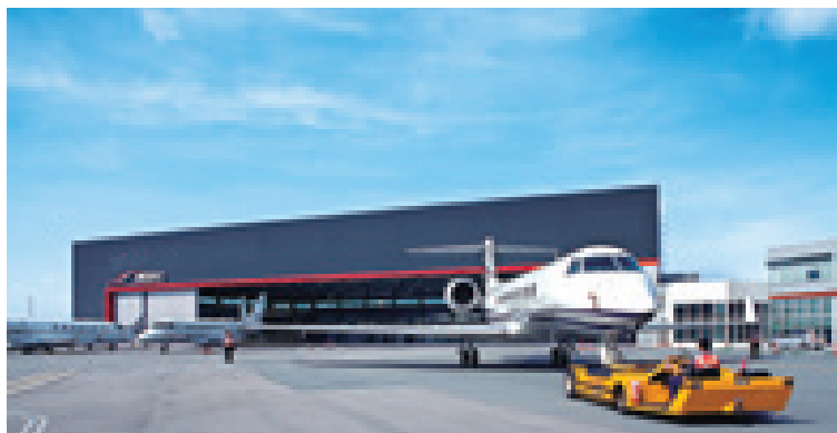
More business aircraft based in the city bode well for the Hong Kong Business Aviation Centre
