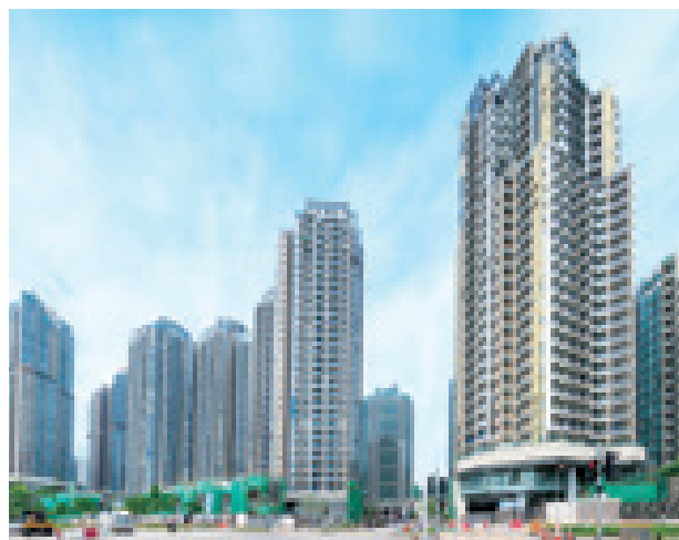
The Wings series of residential developments has spurred energetic growth in the Tseung Kwan O South community
