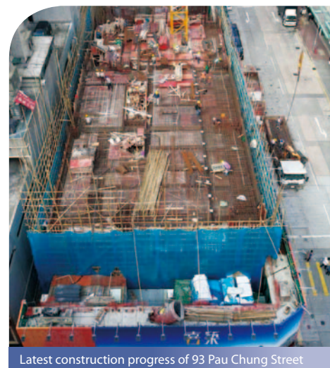
Latest construction progress of 93 Pau Chung Street
