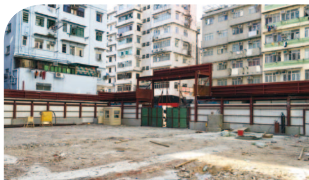
Latest construction progress of Ki Lung Street project
