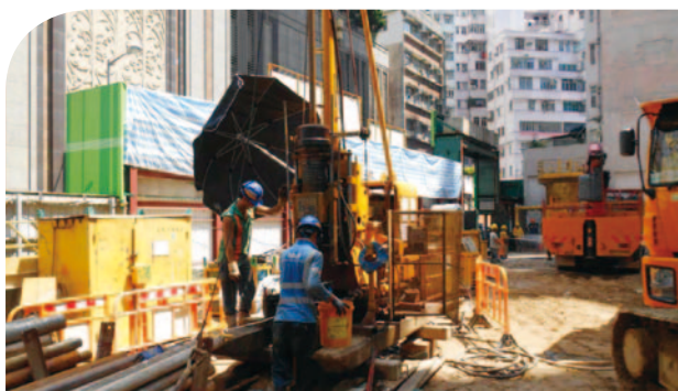
Latest construction progress of Sai Wan Ho Street project
