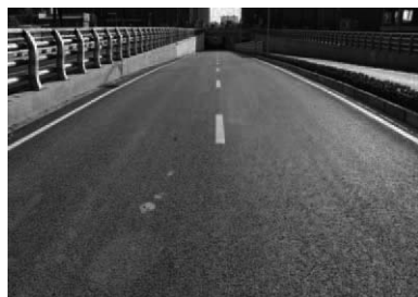
Xiaying Avenue, Ningbo
