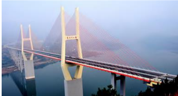
Pengxi River Bridge along the Chongqing-Yibin Expressway.
