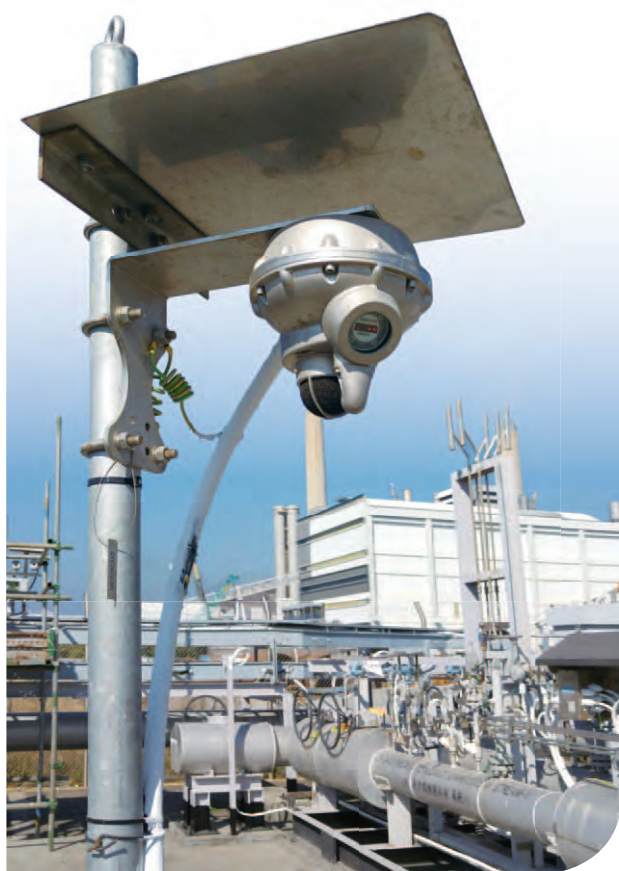
Acoustic sensors installed to enhance the safety infrastructure of Lamma Power Station.
