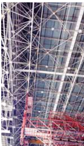
HAECO Xiamen implements ceiling light control in hangars.
