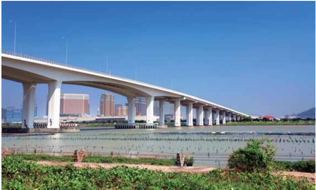
Zhuhai-Macao Lotus Bridge Project
