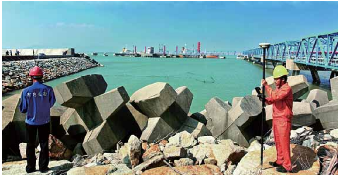
Observation of Ship Channel Subsidence, Gaolan Port, Zhuhai
