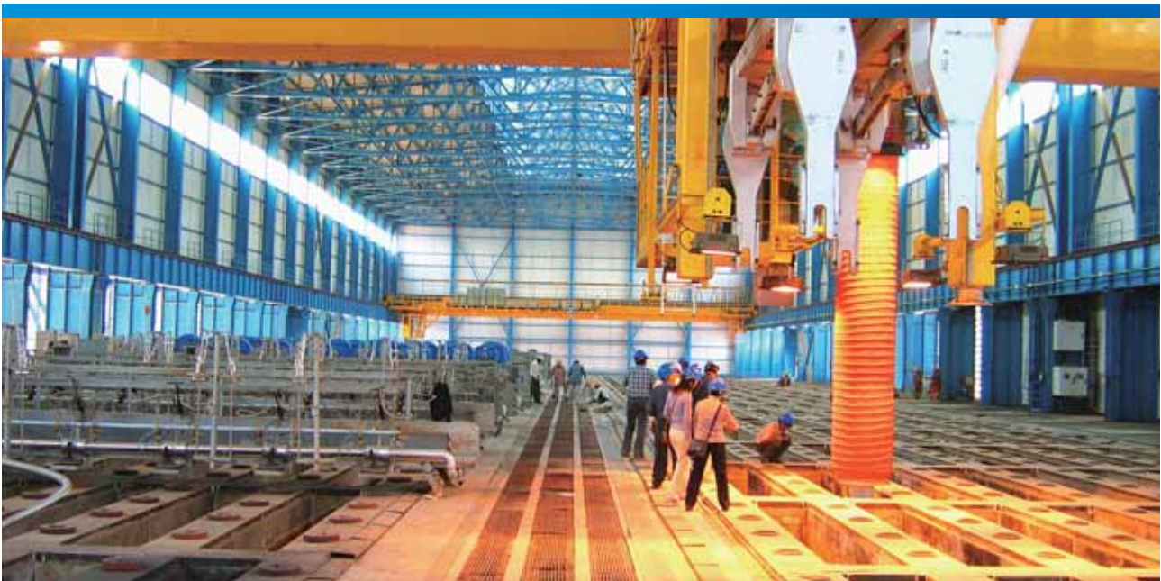
BALCO anode baking furnace in India
