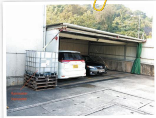
The collected rainwater is used for company car washing, floor cleaning and green area irrigation. "Technical Specifications on Grey Water Reuse and Rainwater Harvesting" published by the Water Supplies Department have provided clear guidance in ensuring the effluent is fit for purpose and poses no undue health risks.
