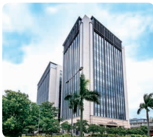
West Kowloon Law Courts Building
