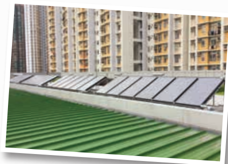
• Solar panels at Sports Centre, Community Hall and District Library Complex in Shatin
