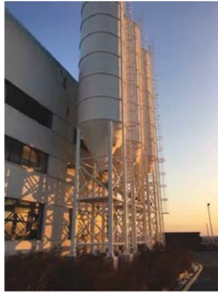
Storage of Material for Pre-Treatment
