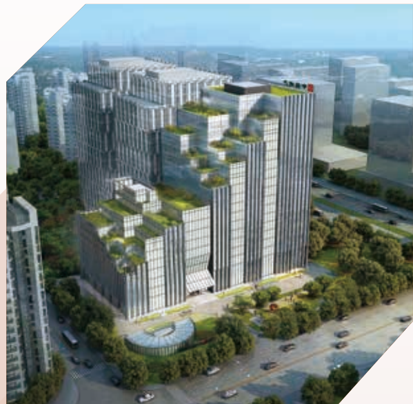
Project JA at Shijingshan District, Beijing
