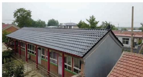
The Application of Hantile on the Roof of a Customer's House in Shunyi District, Beijing 漢瓦應用於北京順義區某用戶住宅屋頂
