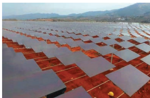
Photovoltaic Agricultural Poverty Alleviation Project in Xundian, Yunnan 雲南尋甸光伏農業扶貧項目
