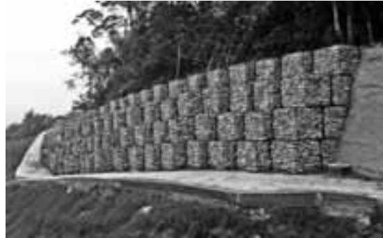
Construction of gabion walls
