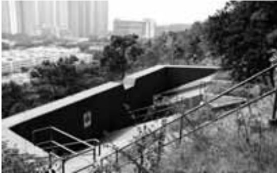
Construction of retaining walls and debris flow protection rigid barriers
