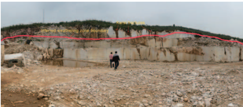
Figure 4-6: Karst and weathering zone occurring in the current open pit
