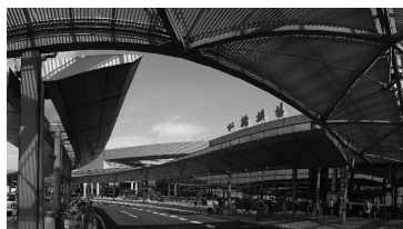
Hongqiao International Airport Eastern Transport Terminal (虹橋機場東 交通中心(公交站區))
