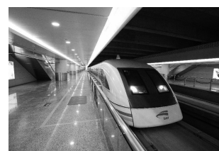
Pudong Airport Maglev Station (磁浮浦東機場站)
