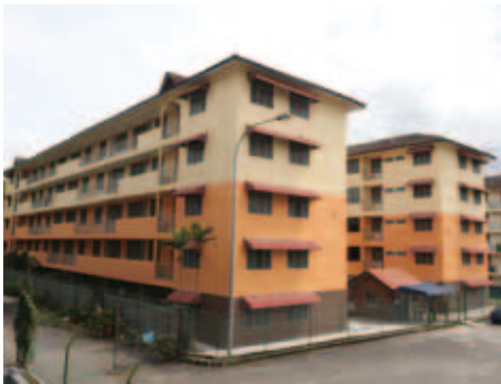
Westlite Pasir Gudang Accommodation
