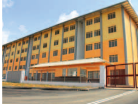
Westlite Senai Accommodation
