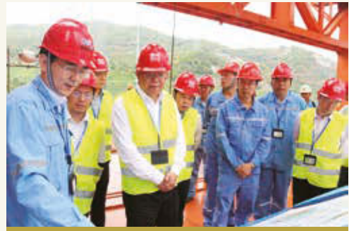
Chairman Wang Jianping conducted safety inspection on Yangjiang nuclear power project
