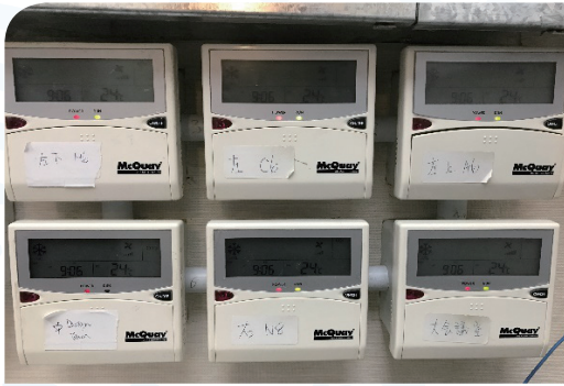
Central air conditioning system to maintain the room temperature at a steady rate 中央空調系統保持室溫穩定
