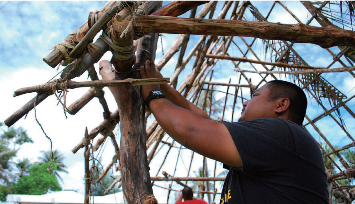
CSR Team rebuilds the Utt during Historic Preservation Month
