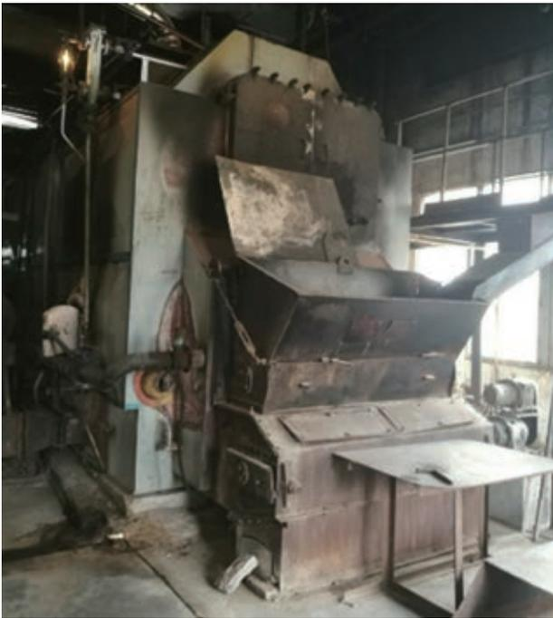
Zhongshan Tungtex burns biofuel in boilers and related facilities to generate heat and steam for ironing in production process and for hot water supply to the staff dormitory. Zhongshan Tungtex has added dust filters and monitors the biofuel boilers' operation regularly to ensure the biofuels are completely burnt. Such arrangements can reduce the emission of ash, smog or dust. Zhongshan Tungtex also uses natural gas for cooking in the staff canteen.
