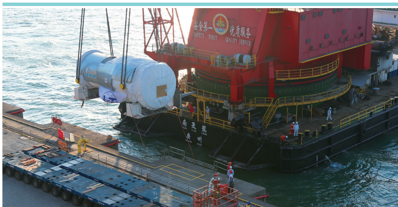
Delivery of major components for additional gas-fired unit at Black Point Power Station
