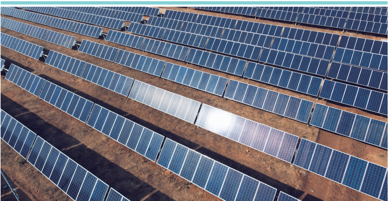
Veltoor, CLP's first solar project in India, is now fully operational
