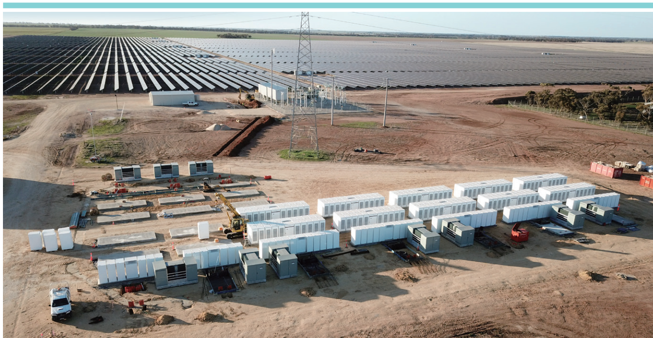
EnergyAustralia has signed agreements to operate two utility-scale battery storage systems in Victoria
