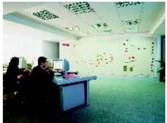
SCADA in Langfang
